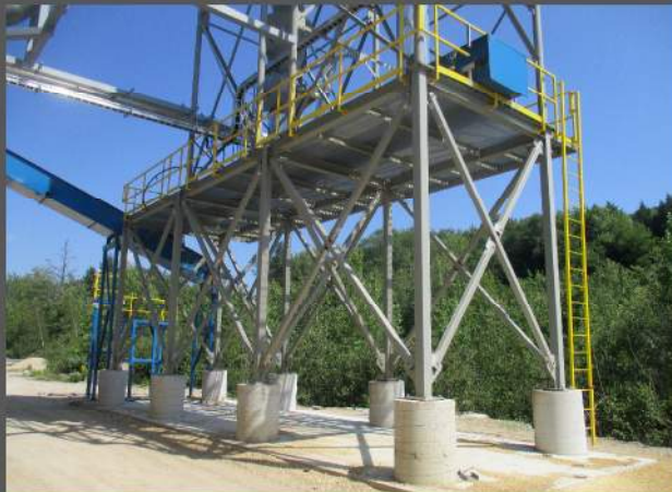
The result of the design is a common braced frame, but the complicated loading conditions made the design challenging.
