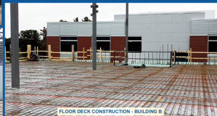
FLOOR DECK CONSTRUCTION - BUILDING B
