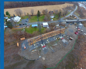
Lifting of timber trusses during construction
