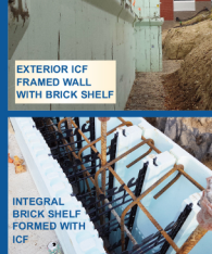
WALL FRAMING 8" ICF WALLS ABOVE GRADE 10" ICF WALLS WITH BRICK SHELF BELOW GRADE
