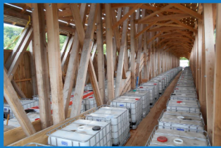
Prestressing of the bridge with 228,000 pounds of water-filled containers
