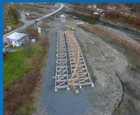
Construction of timber trusses on level ground
