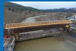
Sliding of the new covered bridge over the new abutments
