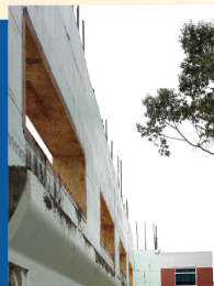
EXTERIOR ICF FRAMED WALL WITH BRICK SHELF
