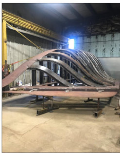
FABRICATION ASSEMBLY (courtesy of DeAngelis Iron Work, Inc)
