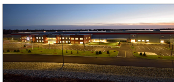
Completed building (courtesy of Greenleaf Construction)
