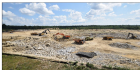
Earthwork and blasting to prepare site (courtesy of Greenleaf Construction)
